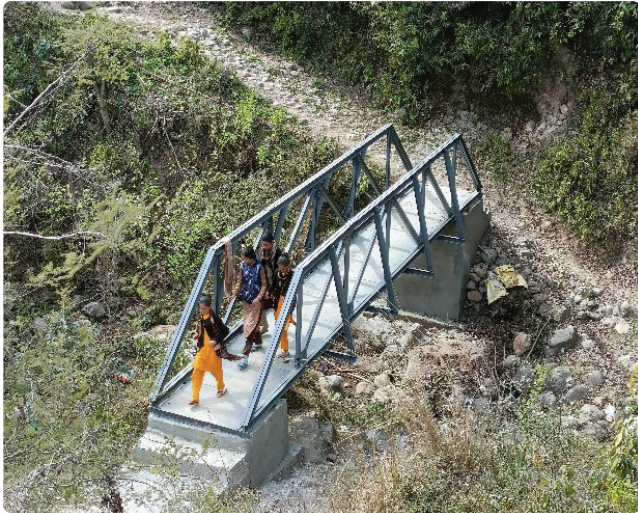
Locals using a footbridge in a village in Raesi District, Jammu constructed through ICICI Foundation's efforts.
